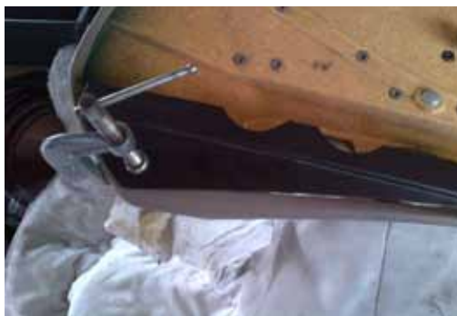
Figure 11 Door panel repair
